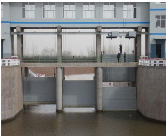
Fig. 1. Flat steel gates application in practical engineering
