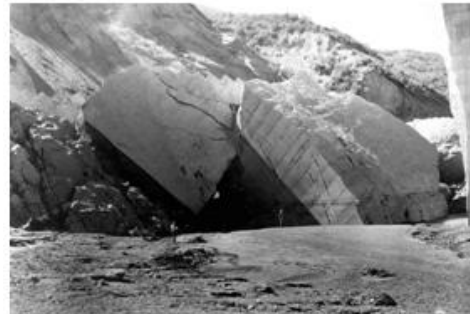
Fig. 2. St. Francis dam break
